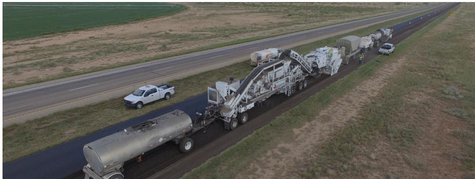
The Indulin family of emulsifiers enables asphalt pavement recycling that reuses 100% of the existing road materials. The process is done in place and without heat. Indulin chemistry facilitates the rejuvenating and replacement of cracked, weathered and potholed roads and highways. This means the process is better for the environment, creates longer-lasting roads, is faster, and less expensive. That's The Ingevity Effect.
